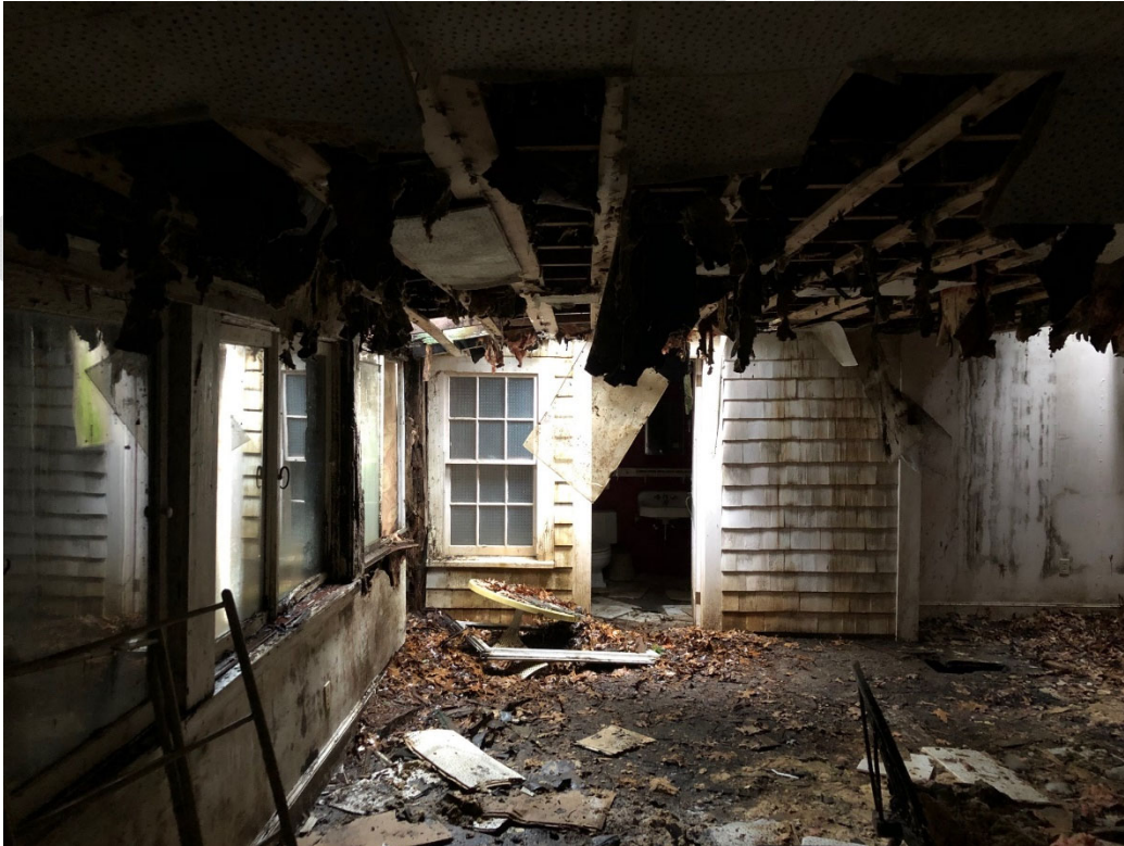
Rear Shed Roof/Ceiling Collapse
