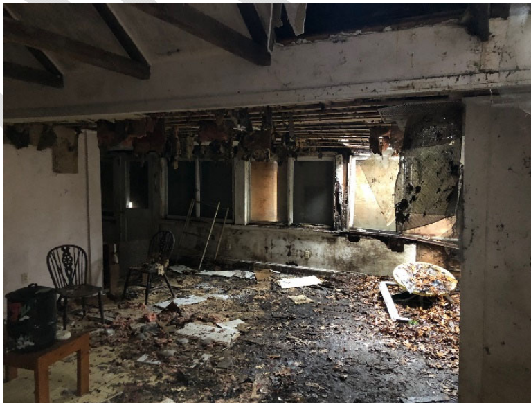
First Floor – Collapsed Ceiling at Rear Shed Roof
