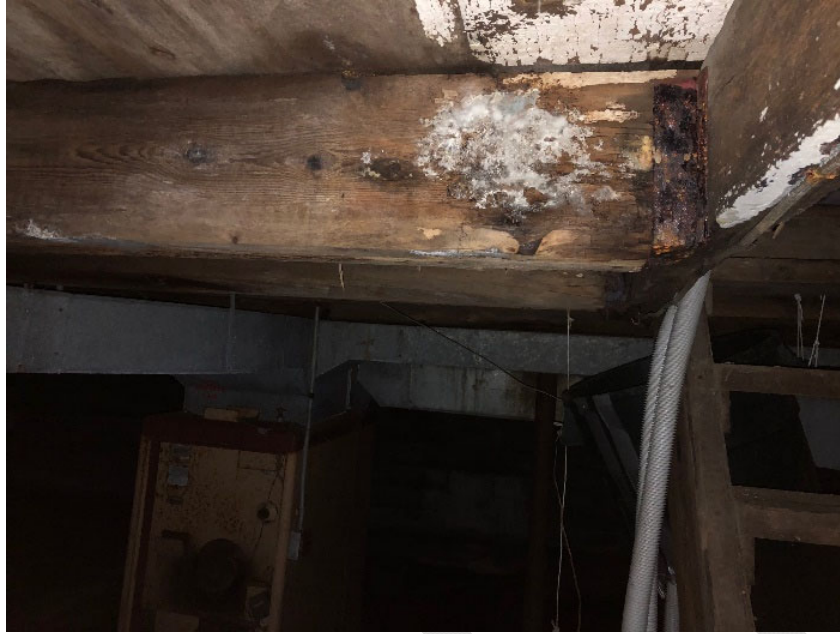
Basement Carrying Beam (Note mold, moisture damage, and corrosion on hanger)
