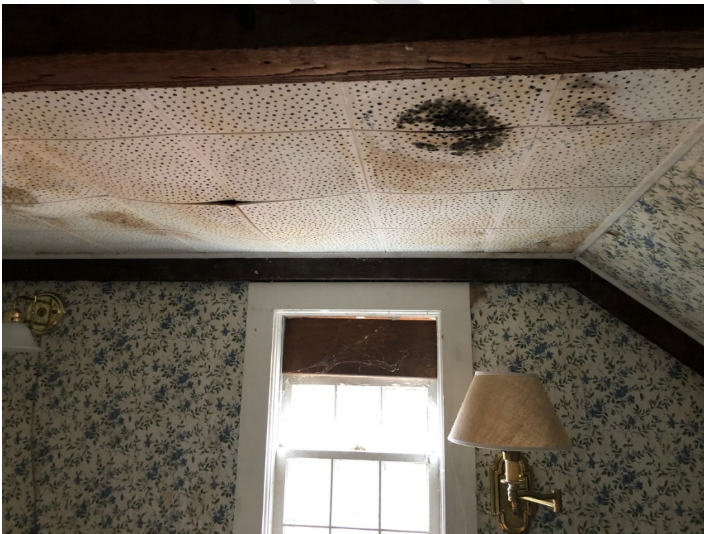
2 nd Floor Ceiling (Note mold and ceiling deflection)
