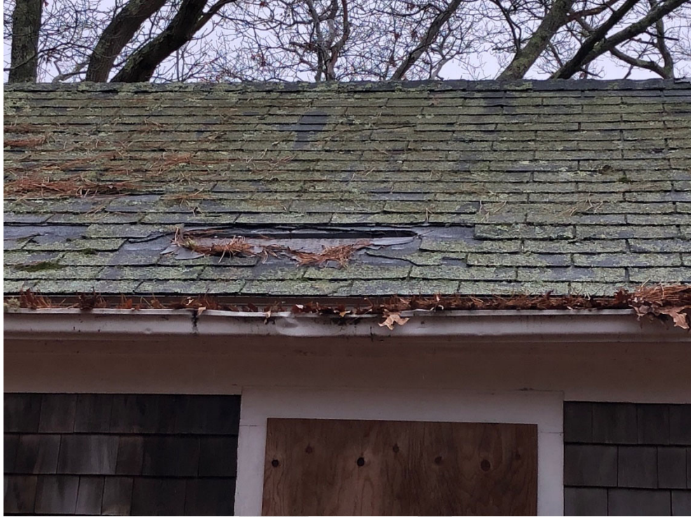
Example of Hole in Roof
