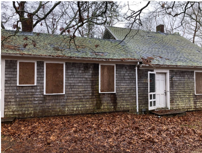
Front Elevation (Numerous holes in roof)
